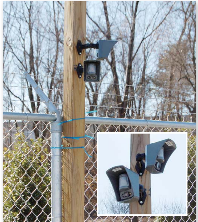
The cameras are easy to set up. In this case, mounting posts are secured to the station perimeter fence with the cameras attached. Since the system is wireless, it can be deployed and re-deployed to suit changing circumstances.
